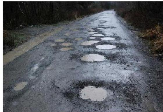
Fig.1. Condition of road with potholes
